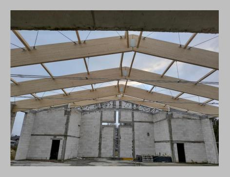
We are rejoicing that the wooden rafters and metal purlins have been installed in the new church building at Biala Podlaska. The next important step is to add the roof, which needs to be in place within the month. The funds required for the roof are \$20,000 and we are praying God will provide during these next few weeks.
